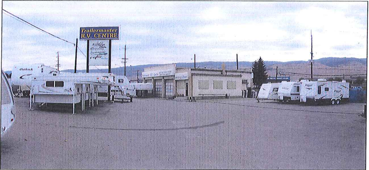
Northeastern perspective of subject site taken from adjacent property to the south.
