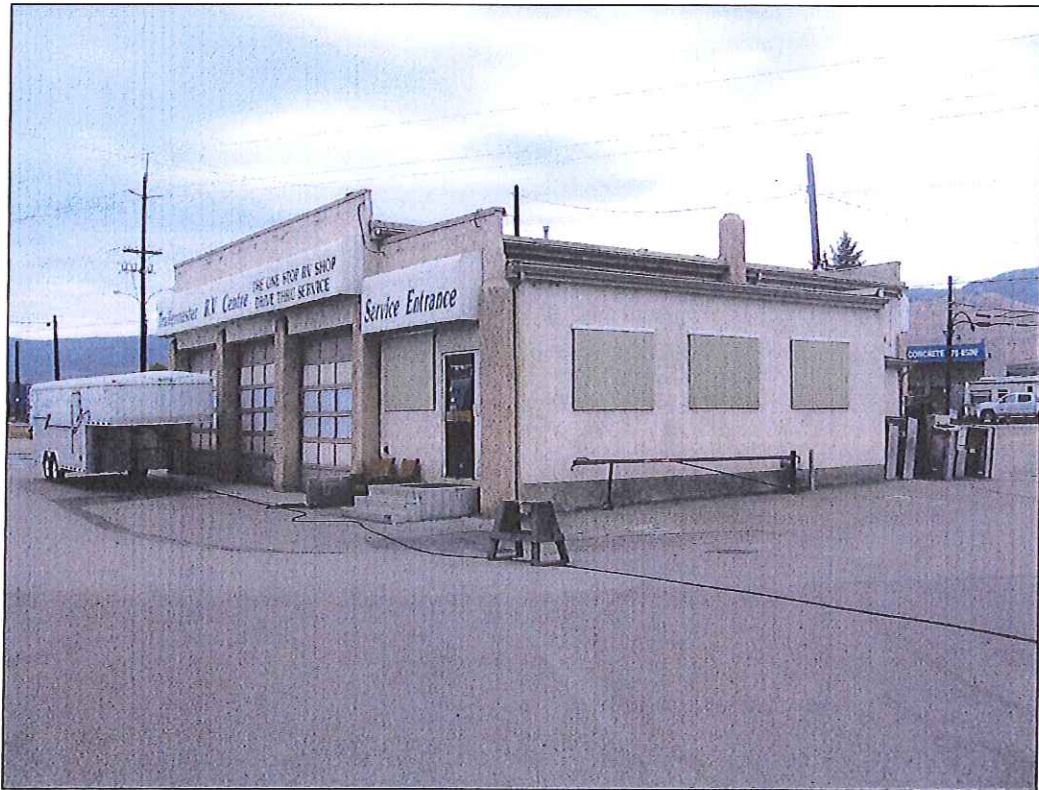
Northeast perspective of western and southern building elevations.
